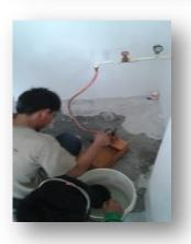
Water Line leak test f 5th Floor 90% Accomplishment
